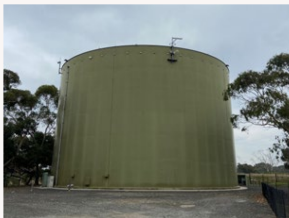
Figure 17. Existing 10ML steel welded water tank at Merrimu
