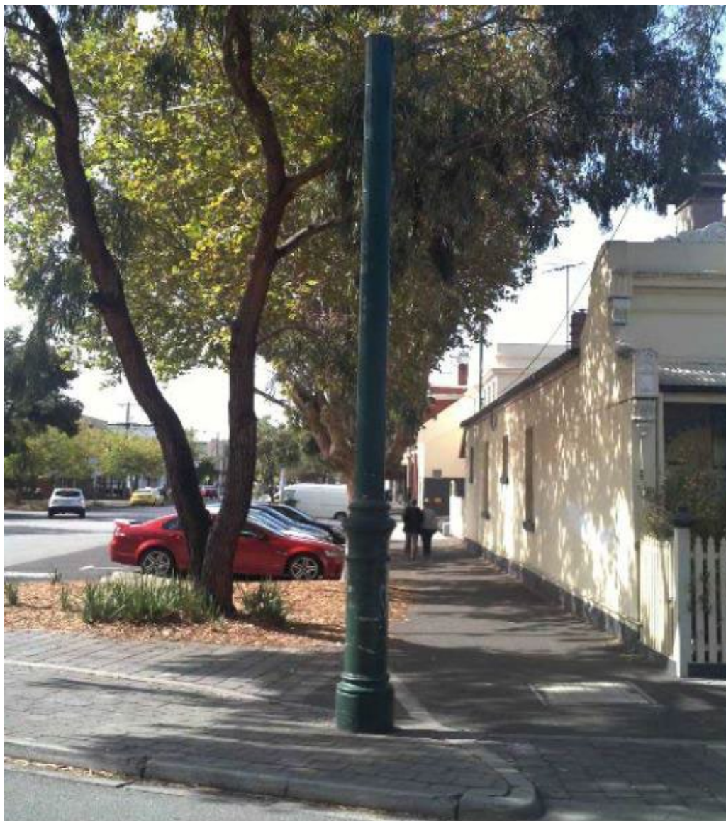
Figure 13: Sewer vent shaft
